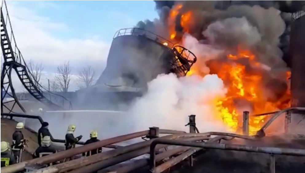
Fire at industrial fuel storage company in Lutsk, via Fox News
